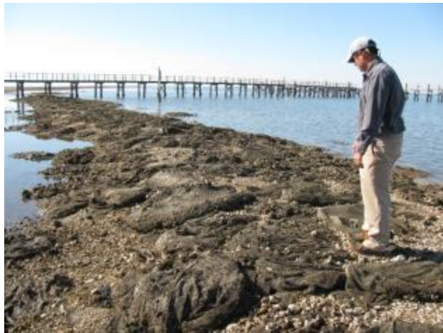
Figure 4. Constructed oyster reef composed entirely of repurposed clam bags on Atsena Otie Key near the town of Cedar Key, FL.
