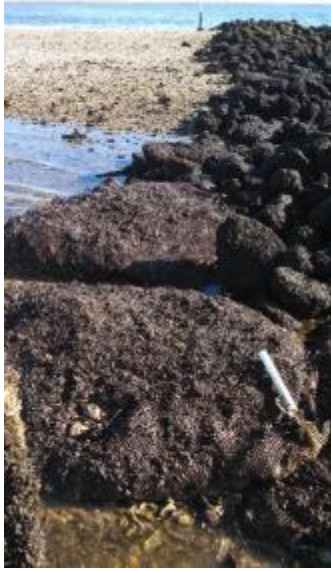
Figure 21. Clam bags as placed on the edge of rock on restoration sites, Lone Cabbage reef.
