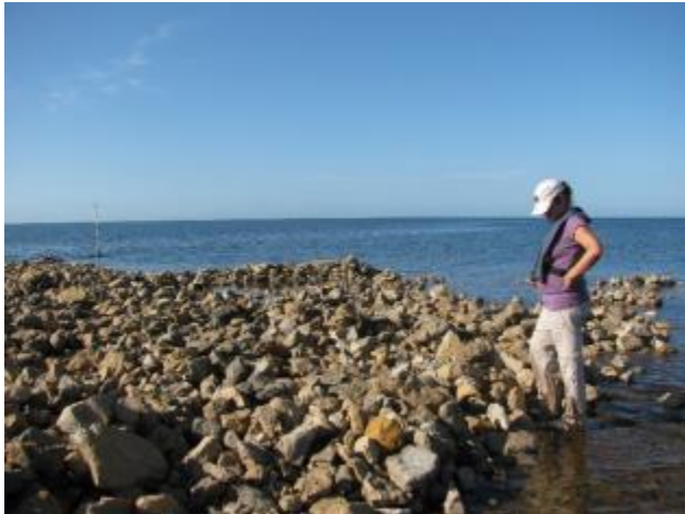
Figure 13. Limerock boulders at low tide on restoration site 1 in the Lone Cabbage reef, approximately 1 week after placement.
