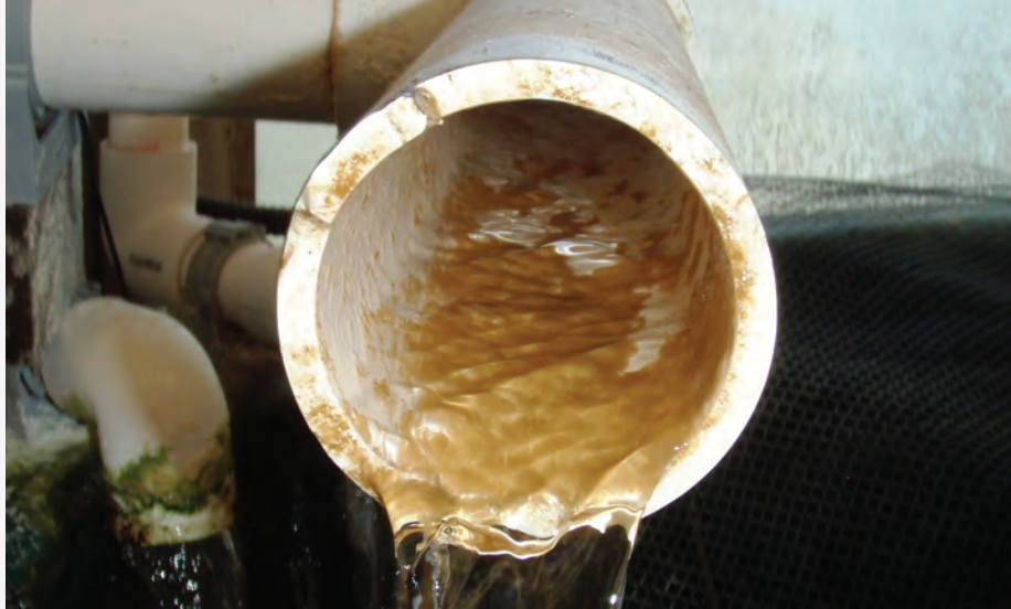
Figure 1: Pipe with a moderate biofilm.
