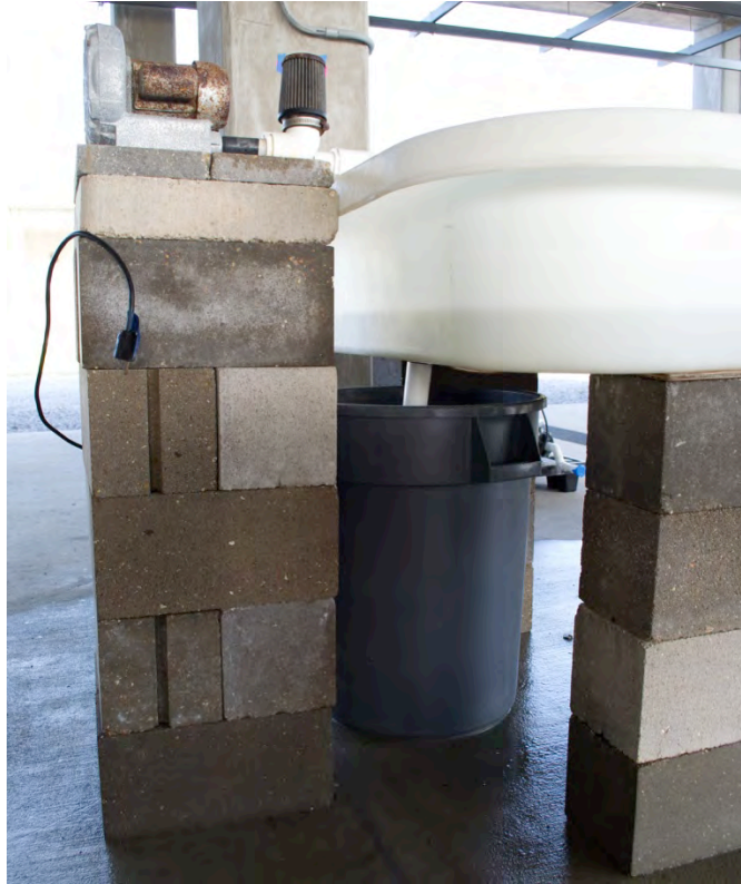
Figure 14. A 35-gallon trash can acts as a reservoir for a setting tank. It is placed under the standpipe drain. Water is then pumped from the reservoir back to the setting tank by a submerged pump and hose.
