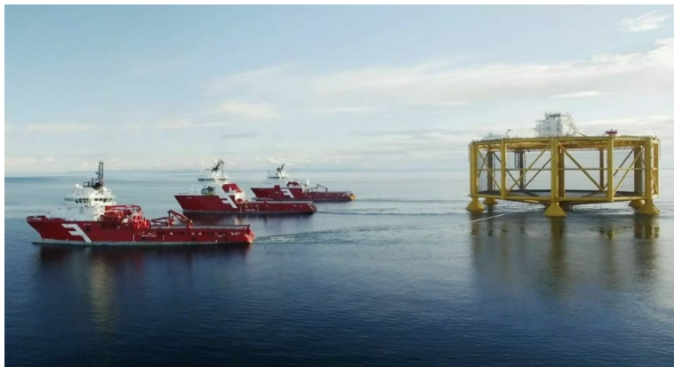
Figure 4.9: Ocean Farm 1™ structure being towed for deployment in Norway 153
