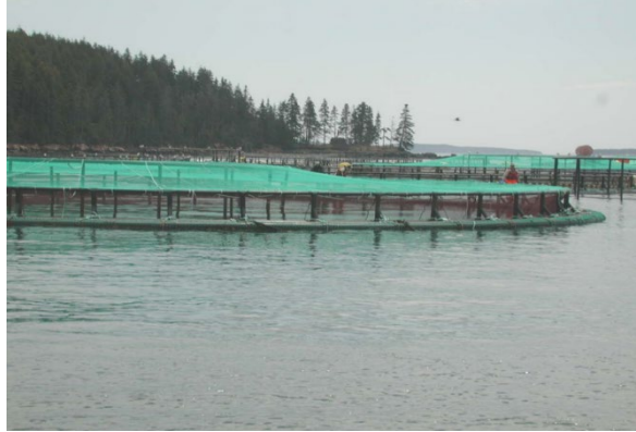
Figure 4.4: Floating salmon net pen off the coast of Maine with green avian predator netting supported in the middle with an HDPE floating support (Photo courtesy of David Bean, NOAA Fisheries).
