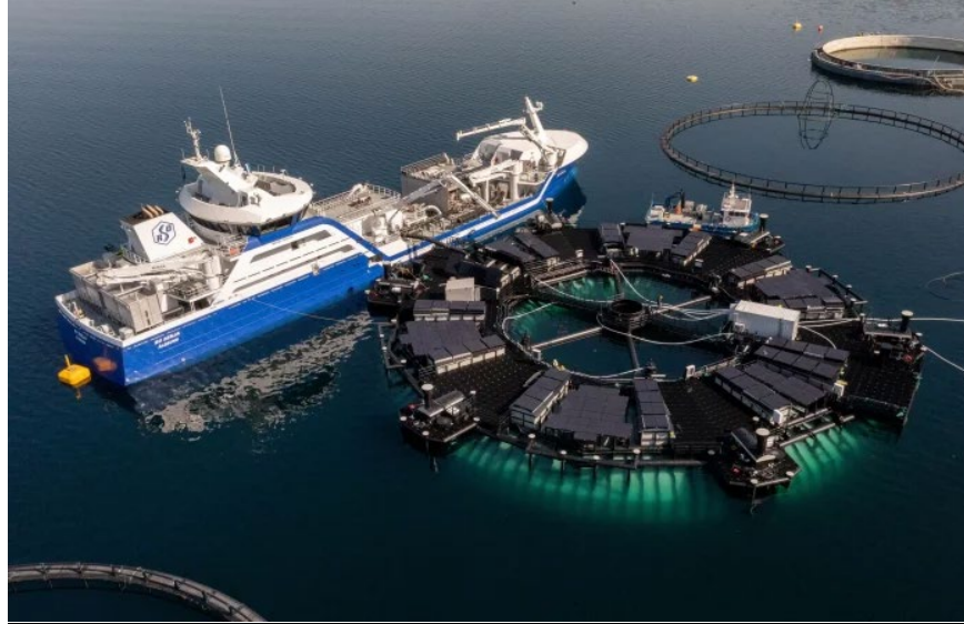
Figure 4.14. The Marine Donut, the donut shaped floating closed containment fish farm operated by the same operators as Ocean 1; SalMar in Norway 159
