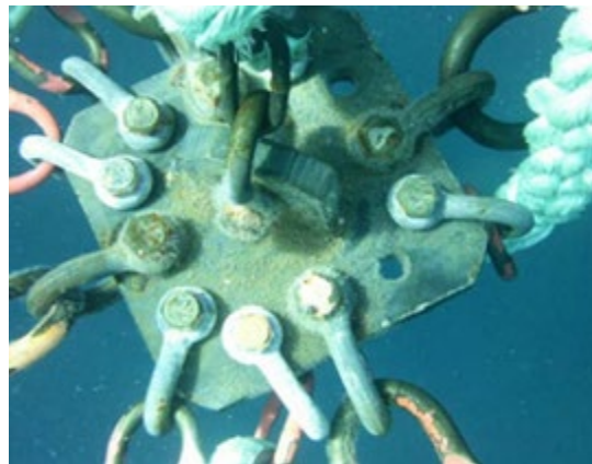
Figure 1.16: Corner plate with multiple shackles connected at various insertion points 28
