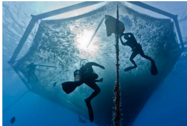
Figure 4.12: Divers service an Innovasea Sea Station™ cage at Blue Ocean Mariculture in Kona, Hawaii (Photo courtesy of Blue Ocean Mariculture)
